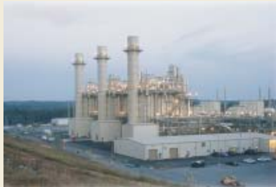
Tenaska's 885 MW Central Alabama Generating Station
