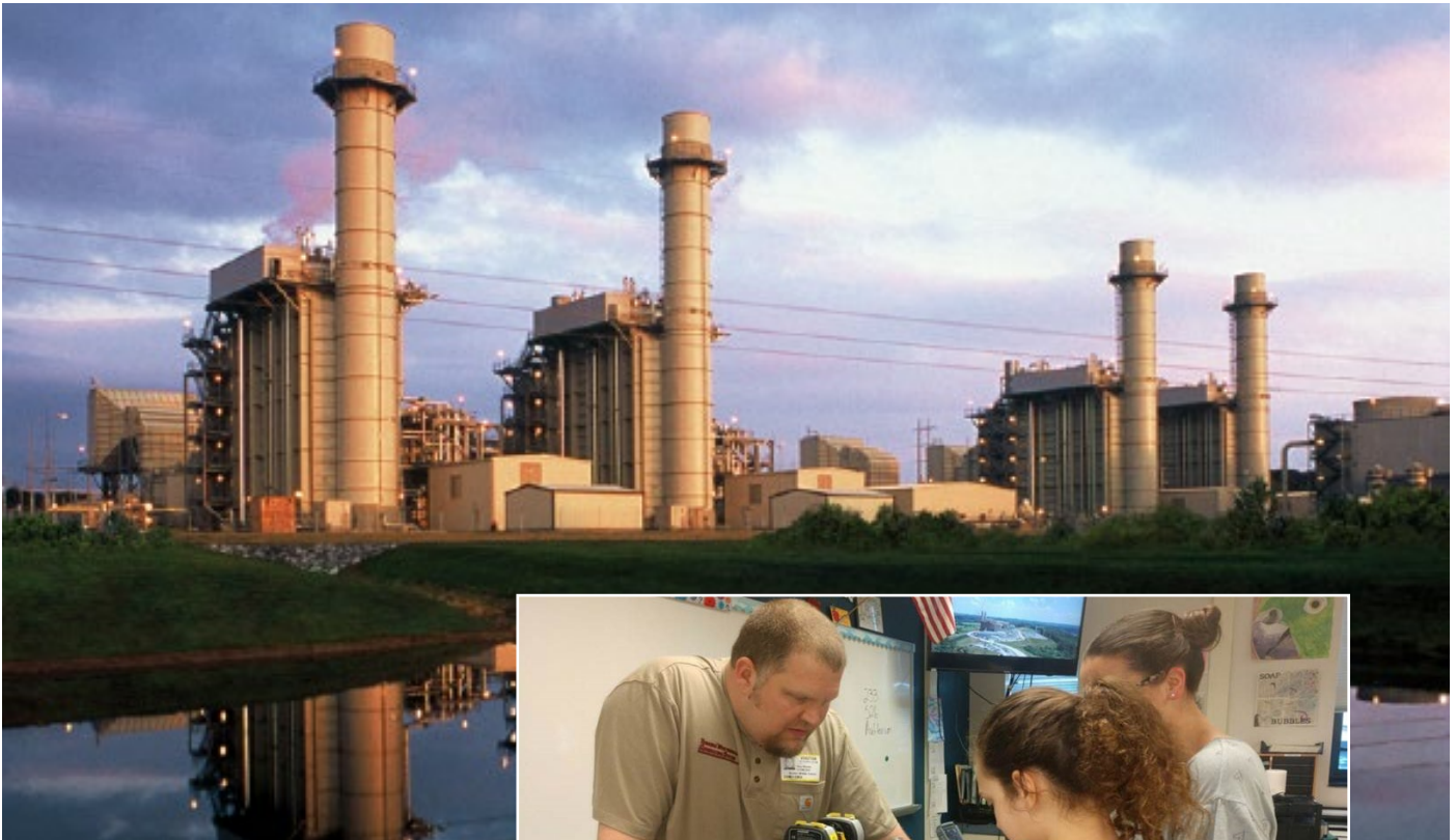
The Tenaska Kiamichi Generating Station near Kiowa, Oklahoma, will provide millions of dollars in tax revenue over the life of the plant. This is in addition to 35 well-paying jobs and various forms of community support, including scholarships to area high school seniors.
